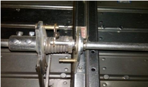
Nailor fusible link and spring
