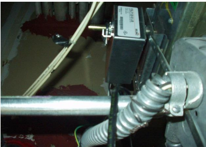
Belimo FSLF direct coupled to shaft.
